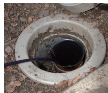
Insert Sleeve in the cleanout
